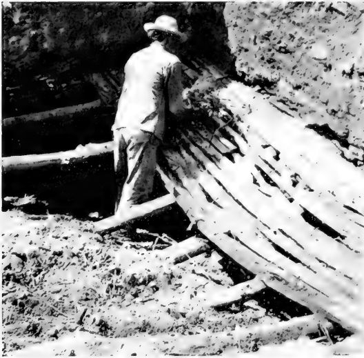
Ceiling and roof construction at Pueblo San Cristóbal. Over the timbers was placed a thicker layer of adobe sufficient to shed the rains
